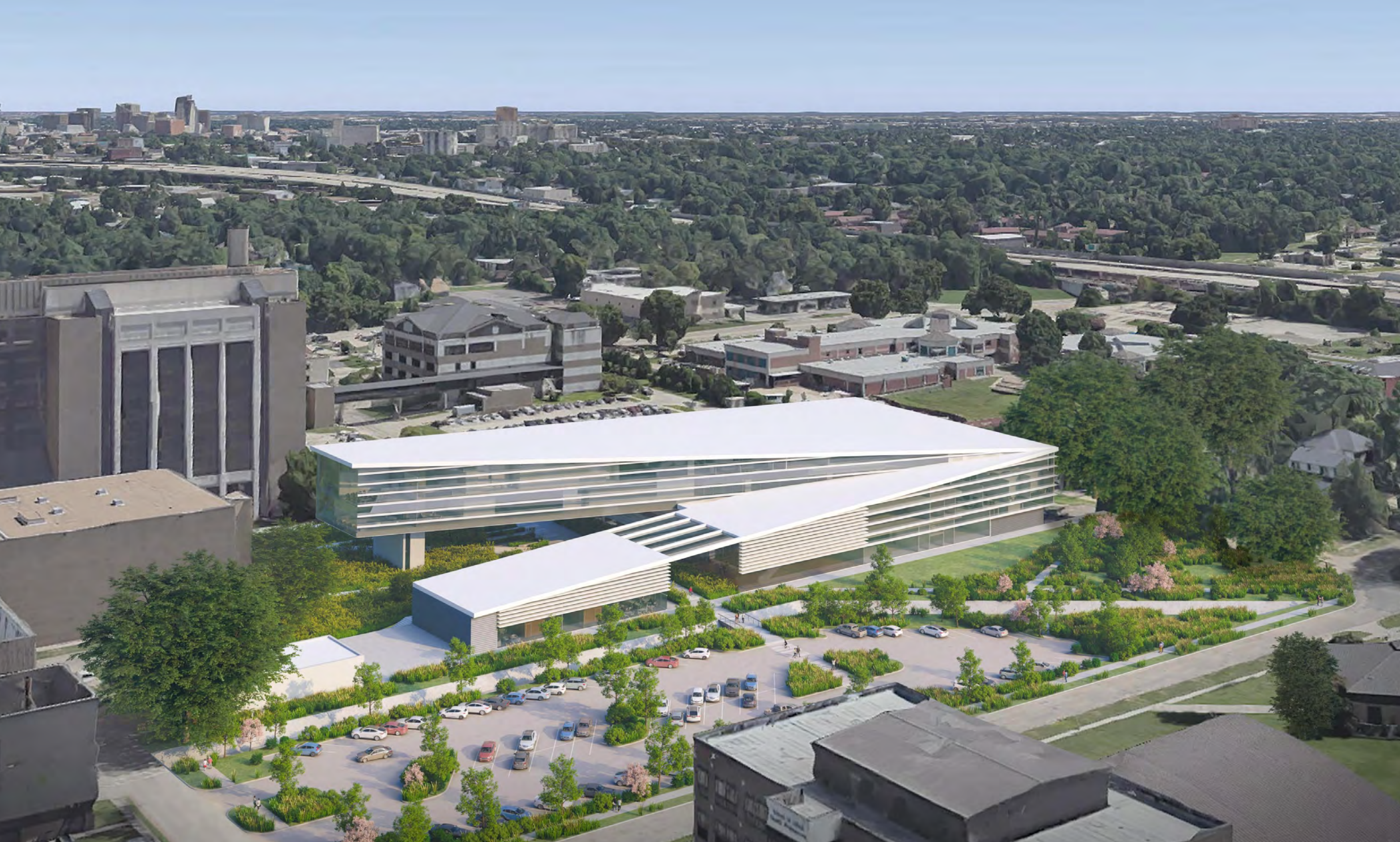
AERIAL VIEW FROM SOUTHWEST
