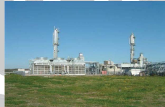
4.6 MW Neptune REG Project, Louisiana
