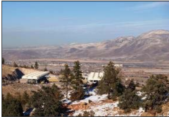
Geothermal Power Plants
