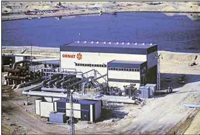
5 MW Solar Pond Collects and Stores Energy - 1982
