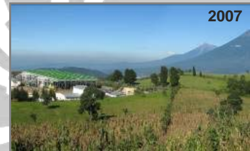
20 MW Amatitlan Geothermal Power Plant, Guatemala
