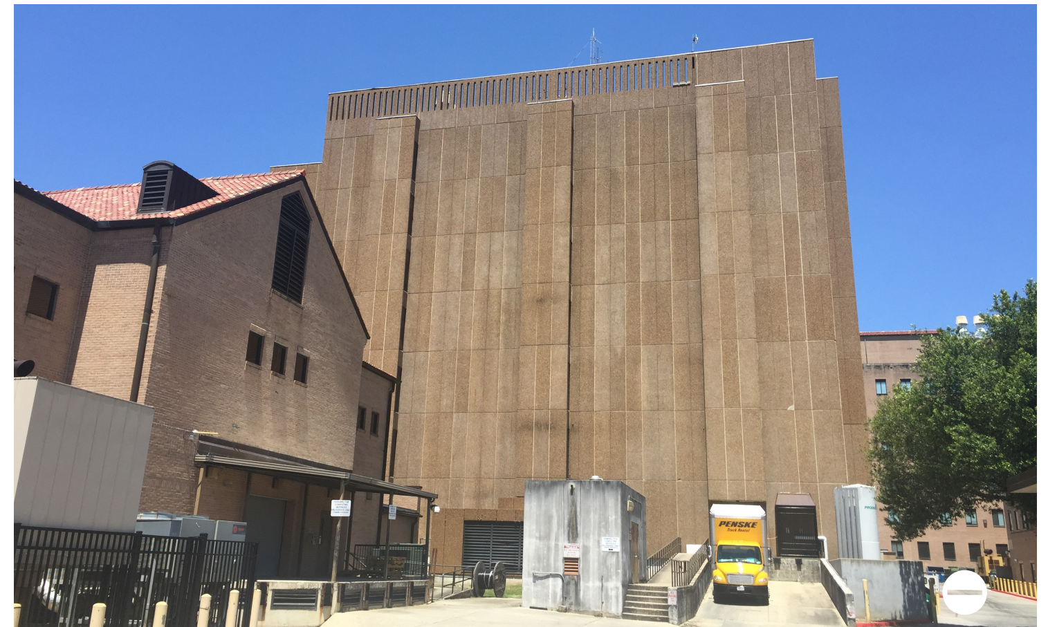
The south facade of Choppin Hall lacks human scale articulation
