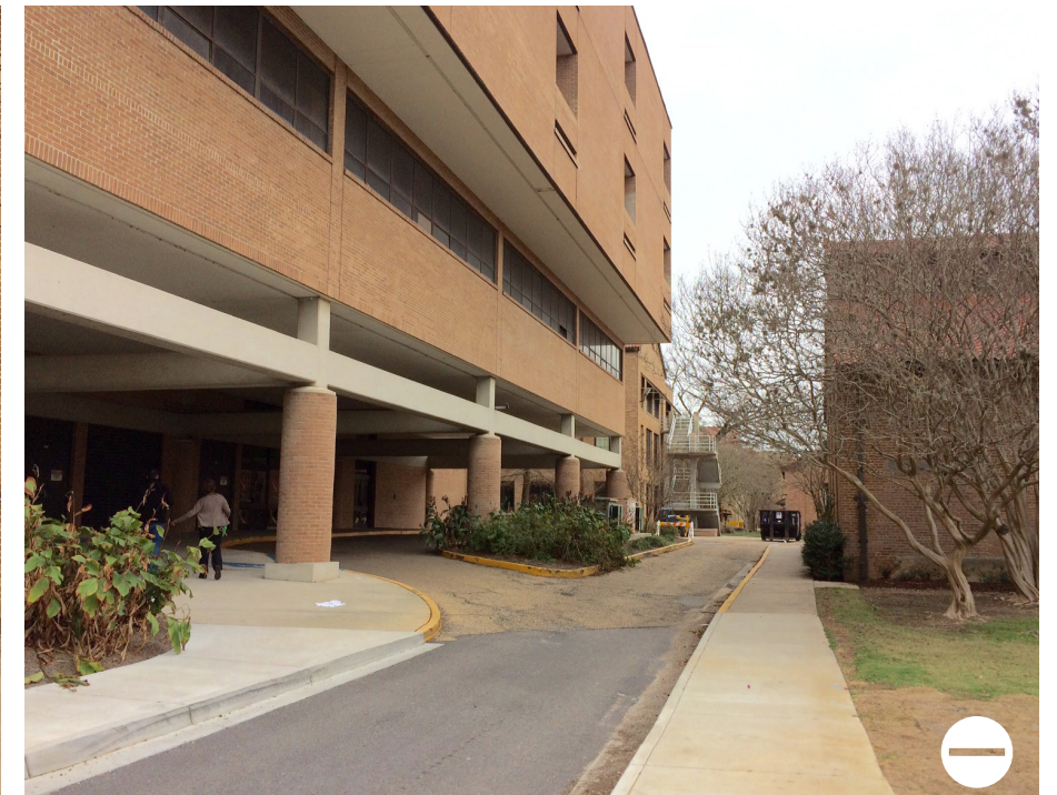
A pedestrian linkage dominated by vehicular and service use
