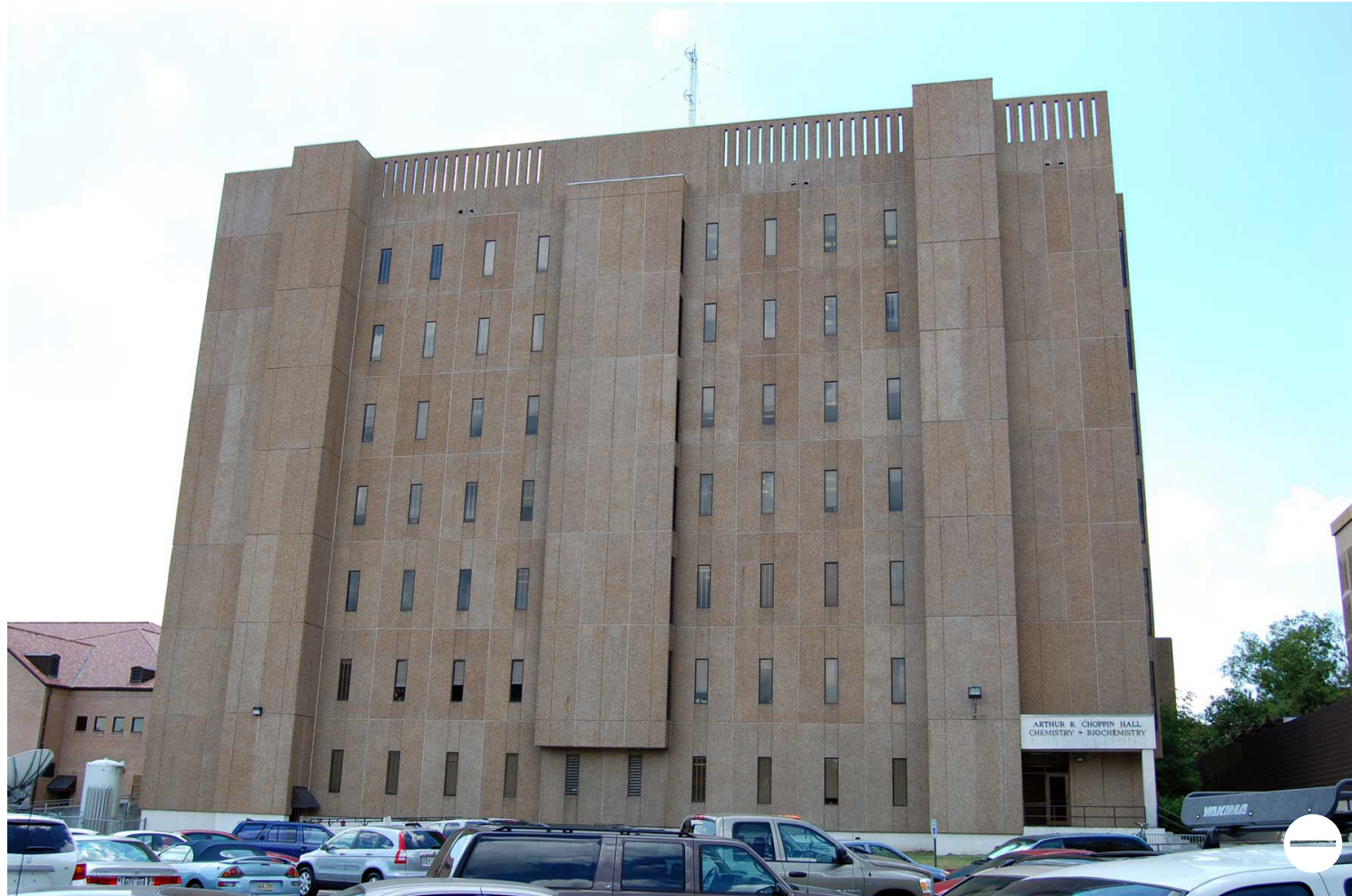
Choppin Hall does not consider daylighting and energy efficiency in its design. The small, unshaded windows contribute to glare on the interior and building orientation does not respond to climate.
