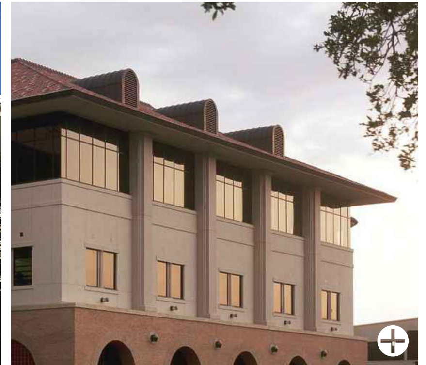
The Emerging Technology Center uses a deep eave to shade high windows, and evenly spaced columns and dormers to relate to historic compositional strategies in a contemporary way.
