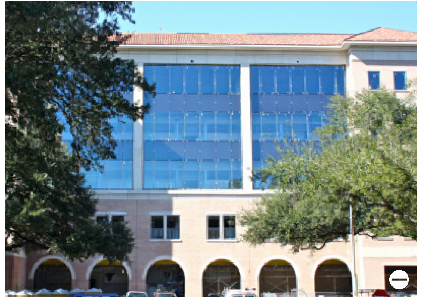
The east facade of the Chemistry and Materials building uses a large amount of unshaded glass, increasing the building's heating load on hot summer days.
