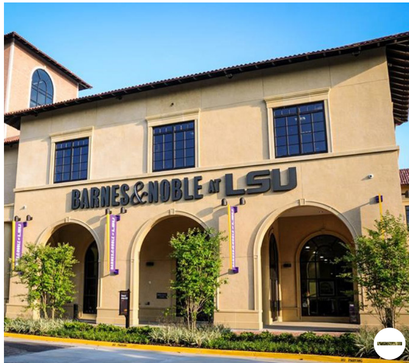
Similarly colored glass and mullions occur at the bookstore. This example could provide a finer grain of human-scale articulation with clear glass, light mullions (like the Student Union shown above right), and / or layering to articulate the facade. This facade will improve as its landscape matures.
