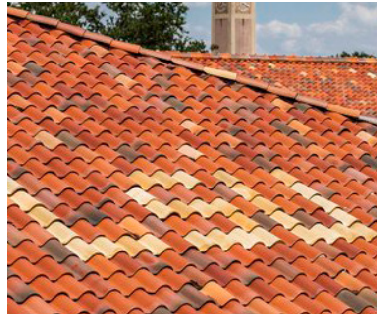
Historic roof material: terracotta tile
