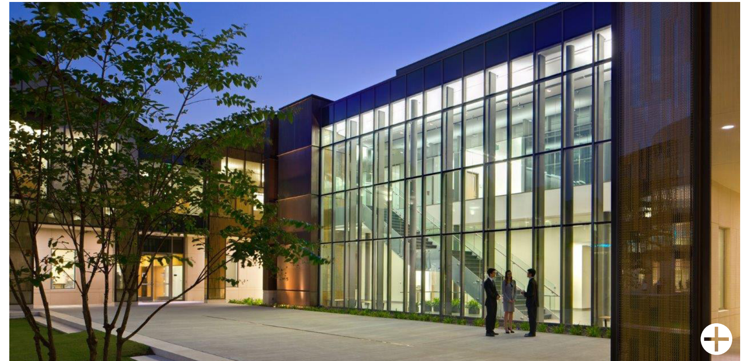
Consider the opportunities for articulation of large curtain wall expanses with vertical and/or horizontal mullion patterns.
