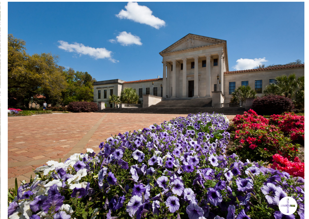
Monumentally scaled architectural conditions are often enhanced by approximately scaled landscape and hardscape elements.
