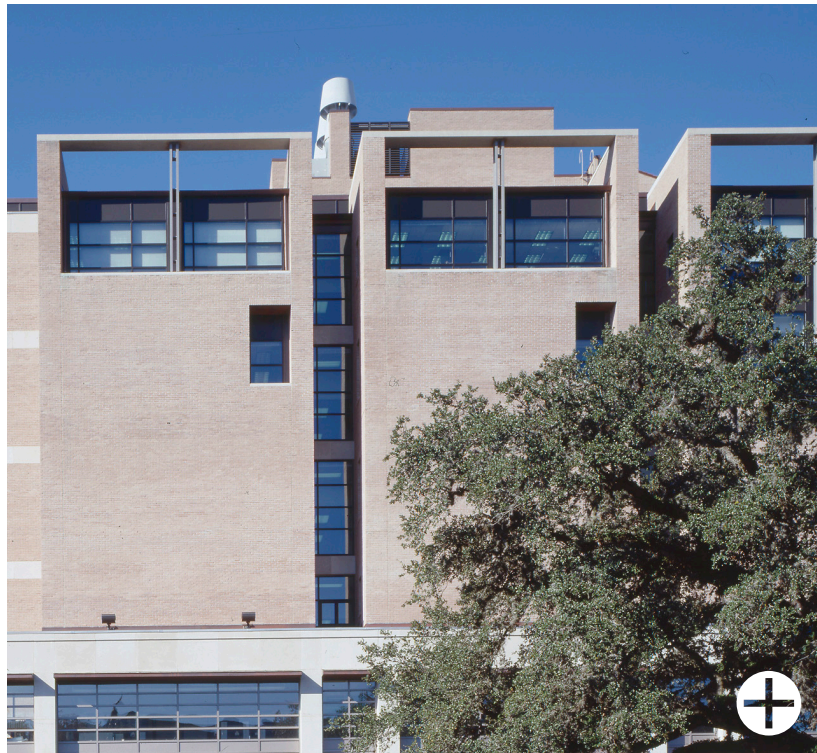
The LSU Life Sciences Annex articulates the building facade with a contemporary eave condition which reinterprets the traditional roof soffits and eaves.
