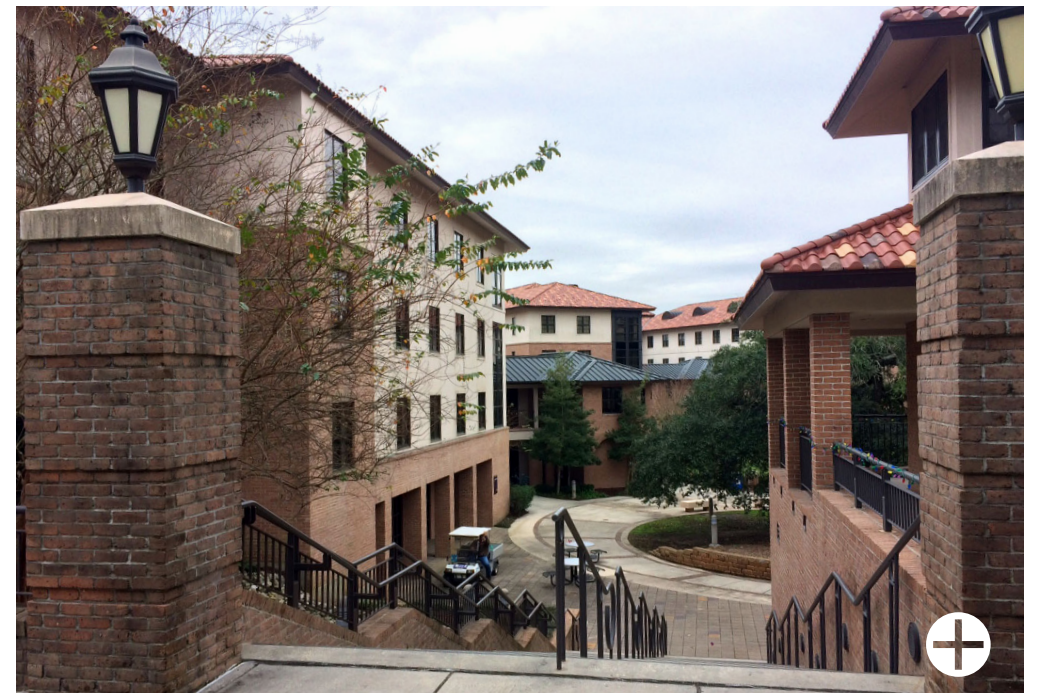
This well-articulated entry to a collection of residence halls utilizes site elements to create gateways and frame views to the courtyard beyond
