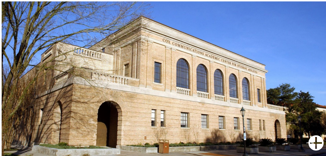
The Gym Armory building top is a well articulated composition without a visible roof or eaves. Ornament here is organized around wall elements to provide a solid, mid-scale texture.
